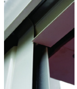
Guide & bottom rail interface
