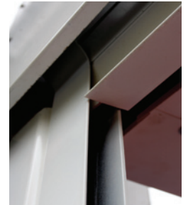
Guide & Bottom Rail Interface
