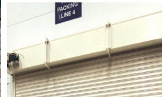
Hood (coil casing) & support brackets
