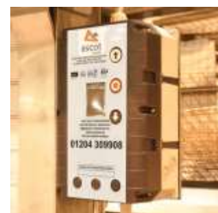
direct drive control panel
