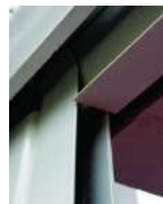
Guide & bottom rail interface
